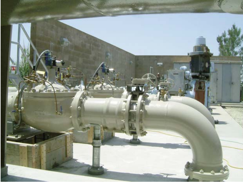
Combination Surge Relief Valves with programmable closing time feature
